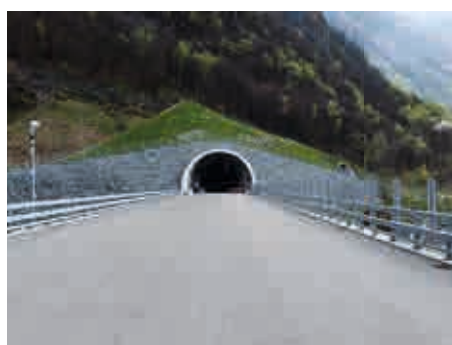
Abb.6: Nordportal Tunnel San Fedele, Roveredo GR
