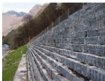
Abb.7: Nordportal Tunnel San Fedele, Roveredo GR
